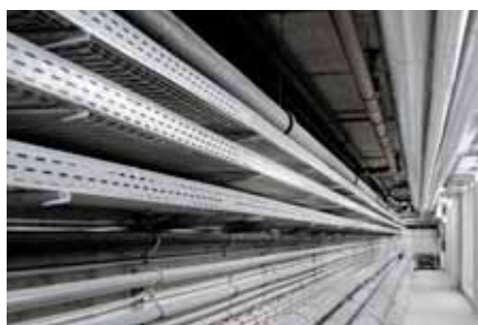
Cable trays, pipe installations
