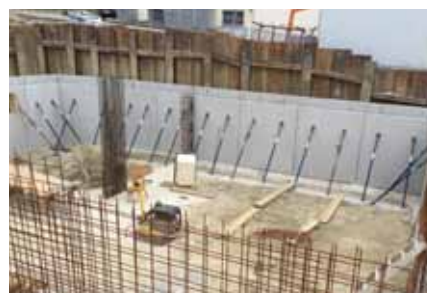
BTS M: Inclined supports / site facilities
