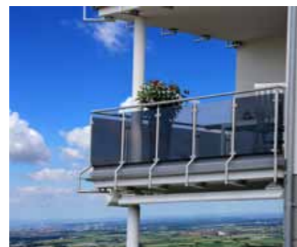
Balcony rail fastening
