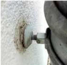
The anchor was pushed too far into the insulation and the hole was ugly sealed.
