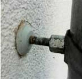
After a short time the galvanized hanger bolt shows already corrosion.
