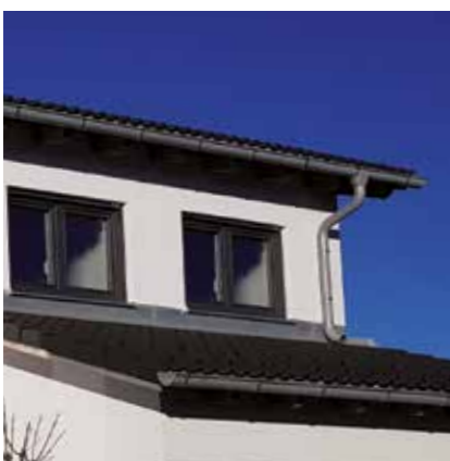
Application wall connection profile above garage
