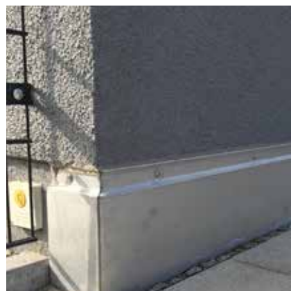
IPSD installed with plumber screw
