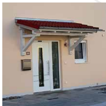
Application wall connection on canopy
