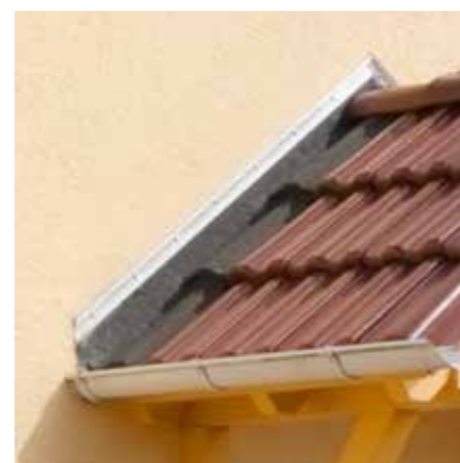
Application wall connection profiles
