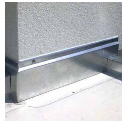
Application wall connection profile
