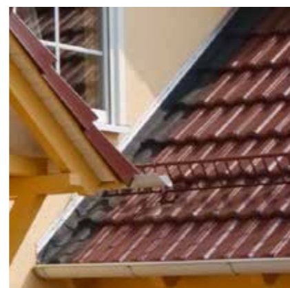
Application wall connection profile
