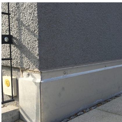
IPSD installed with plumber screw
